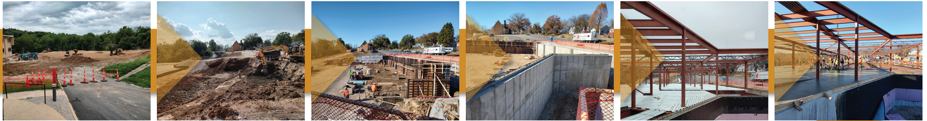
Front construction progression from September 2023 to April 2024. (Photo by Ken Stout)
